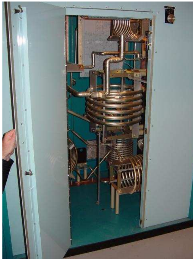
Figure 3.18: High power inductors formed from hollow tubes.
